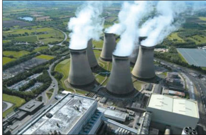
Three of the six generating units at the Drax Power Station, the UK's largest generating facility, are being converted to burn biomass, much of it in the form of wood pellets produced in the US, in place of coal. Each converted unit will provide enough renewable electricity to meet needs of more than 1 million homes.
